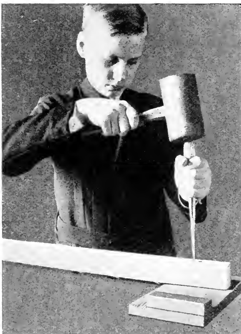
Fig. 19. Position of Chisel and Mallet for Mortising.
